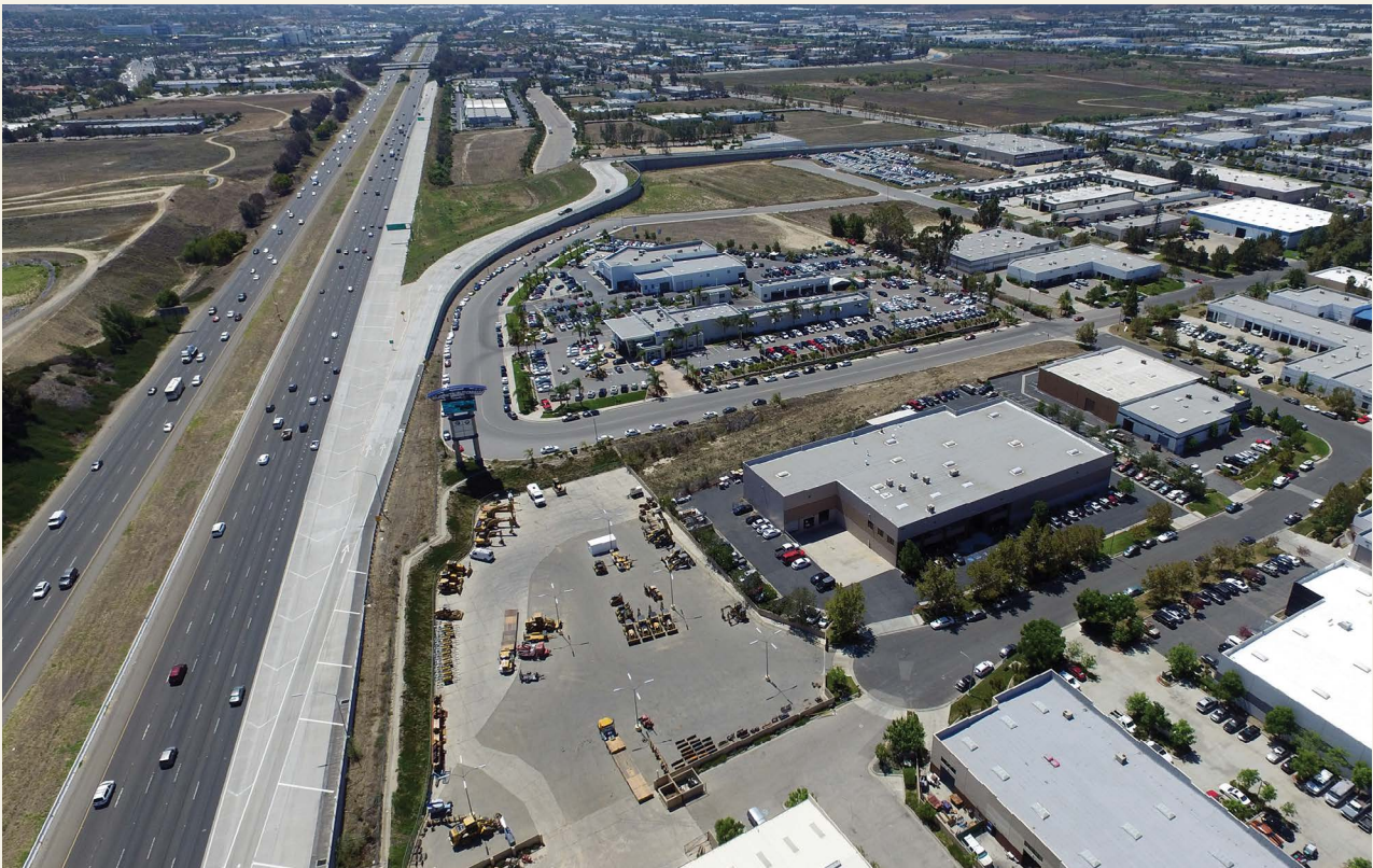
French Valley Parkway off-ramp project
